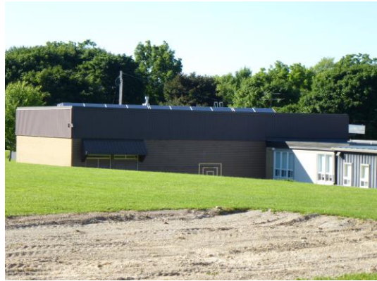
10 kW Rooftop Solar System Brussels Business & Cultural Centre
