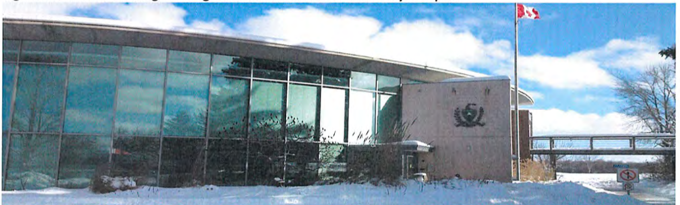
Figure 3: Photo of existing building known as the Health and Library Complex
